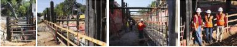
Moffat Pipe, Inc. (MPI), based in Wake Forest, N.C., currently is in the process of installing 320 linear ft. (97.5 m) of 5 by 10 ft. (1.5 by 3 m) cast-in-place concrete culvert pipe through the neighborhoods of Raleigh, N.C.
