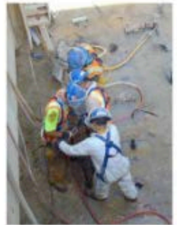
Workers in the microtunnel launch pit at Hodges Street
