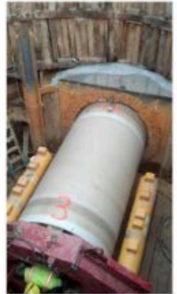
Microtunneling at New Burn Avenue
